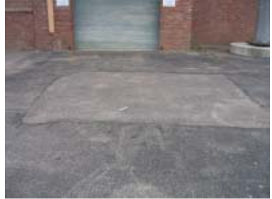
Patched asphalt where Hunley crew were found.
